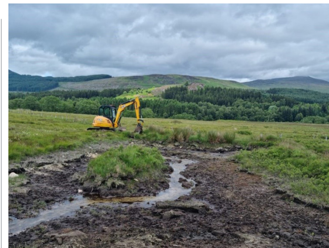
Wader Scrape being installed at Glenshero Estate
