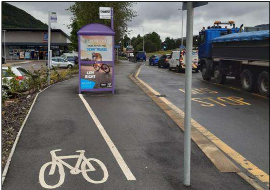
Figure 3.6: Cycleway (and Bus Stop) Along A82 Adjacent to Retail Park
