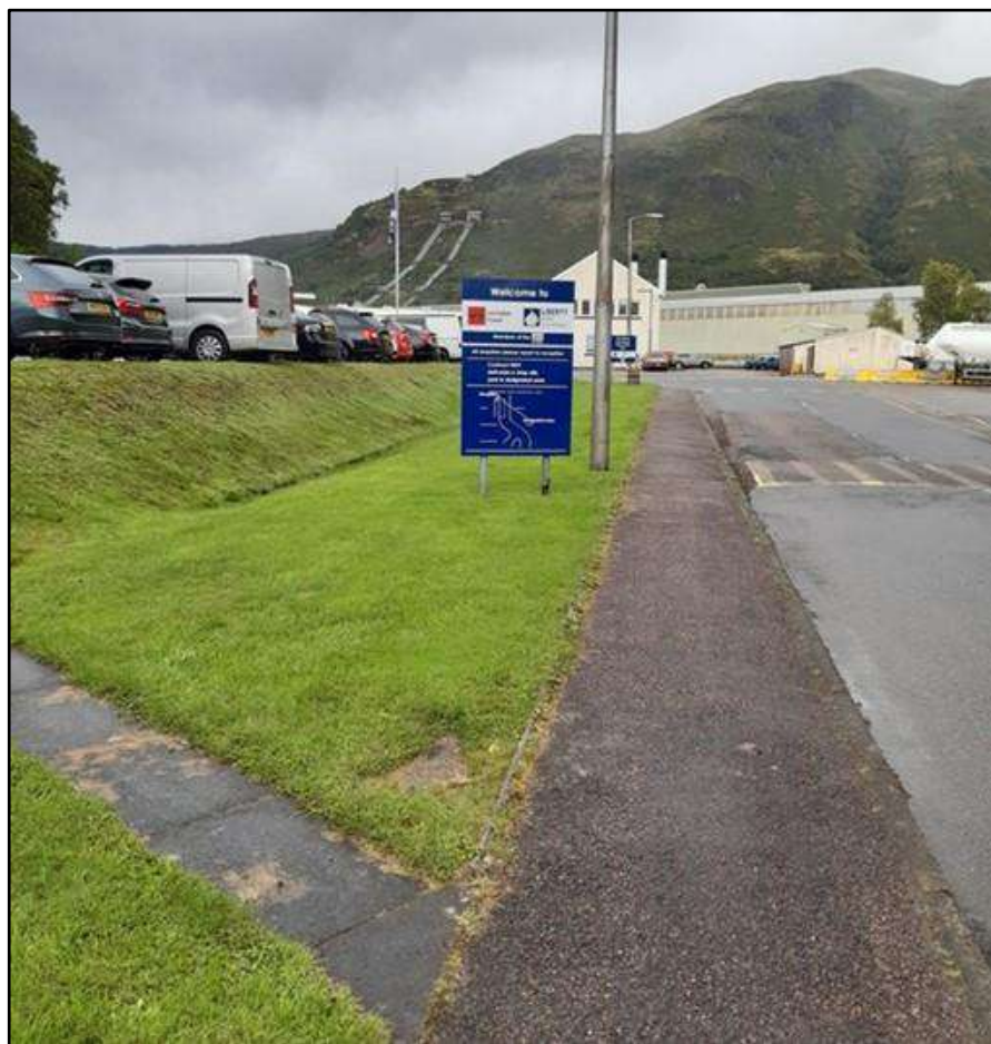
Figure 3.2: General Characteristics of Access Road Footway
